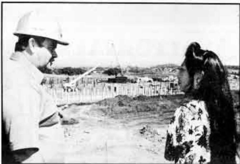
HIGH SCHOOL ON HIGH — Susan Scofield, the administrator selected to open King Kekaulike High School when it is ready for its first freshman class next fall, tours the Five Trees site in Kula with construction supervisor Tim Gatschet.
